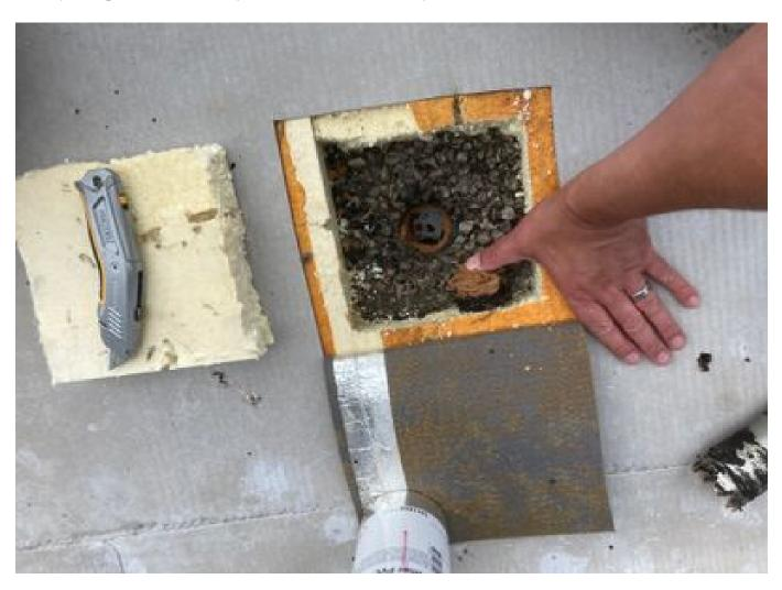
**Core Sample Moisture Result:** Moisture was found in the roof build up above the structural deck. Good roofing practice dictates that the existing roof build up should be stripped.
