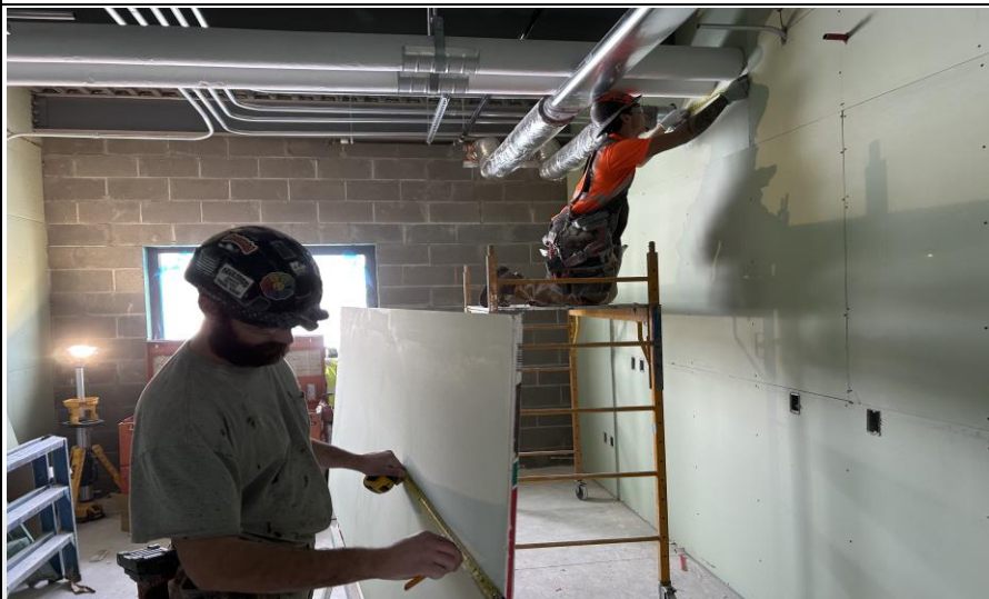
BEK Clear Dormitory Project
