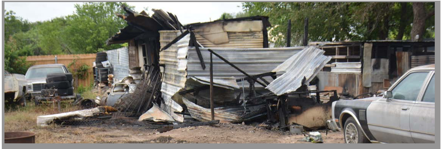
An early-morning fire on Monday caused this recreational building to collapse. One person died from the incident.
