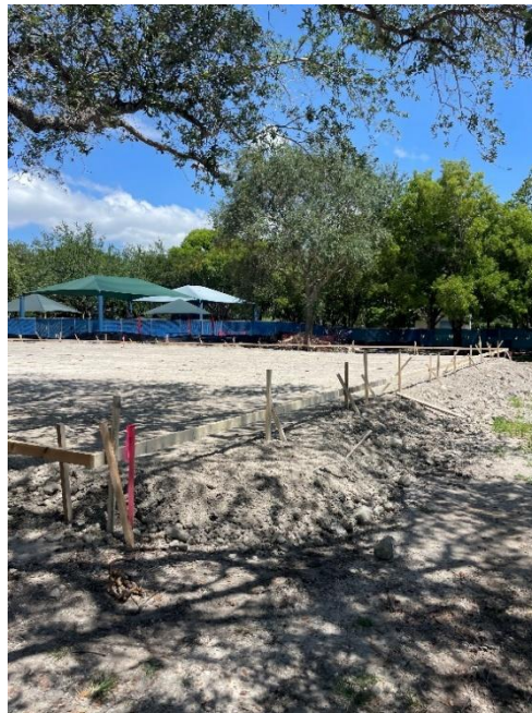
Frame for the pouring of the foundation slab
