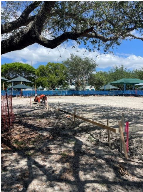
Frame for the pouring of the foundation slab
