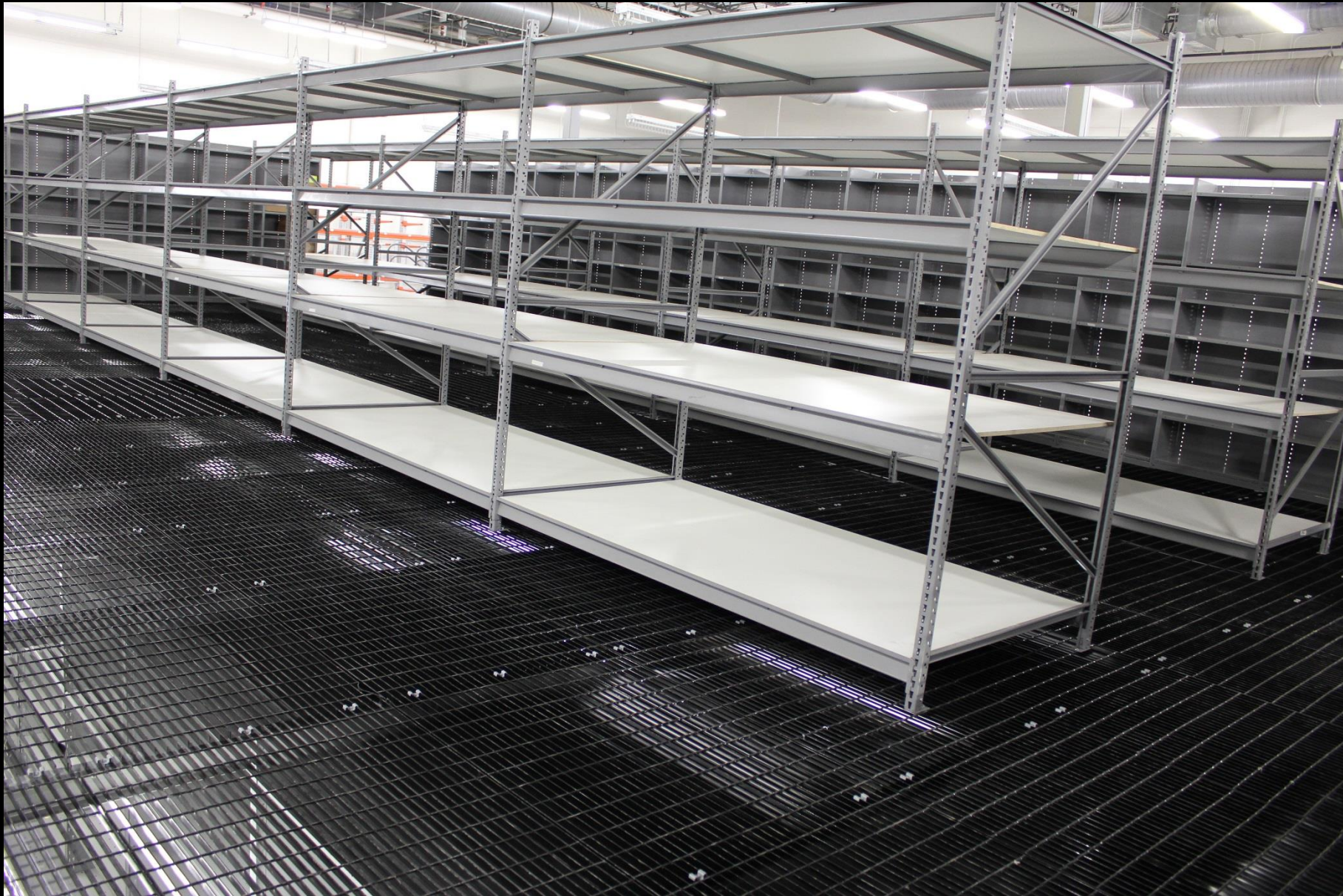
Steel Shelving Supported Catwalk/Storage System
