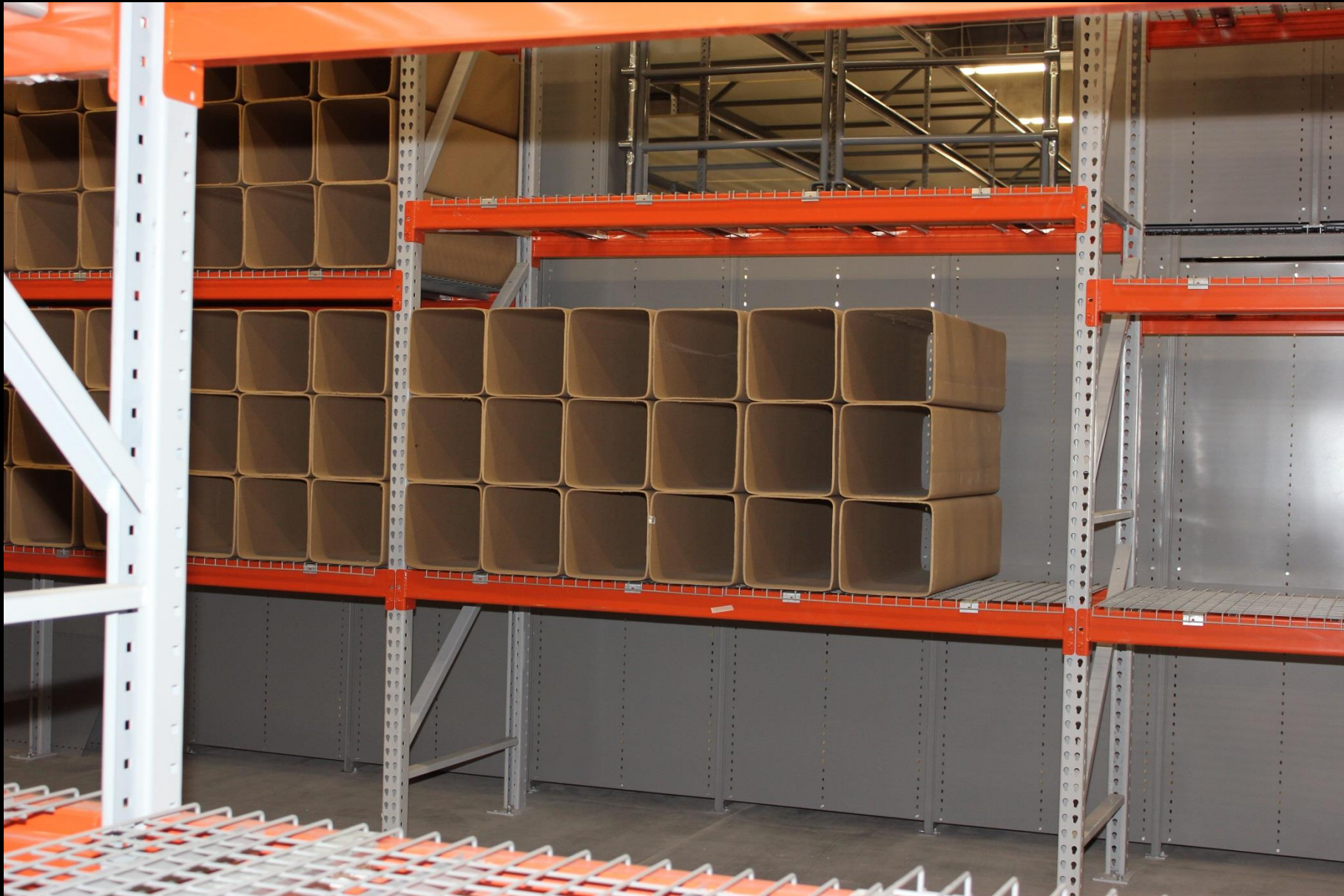
Custom Pallet Rack Storage System
