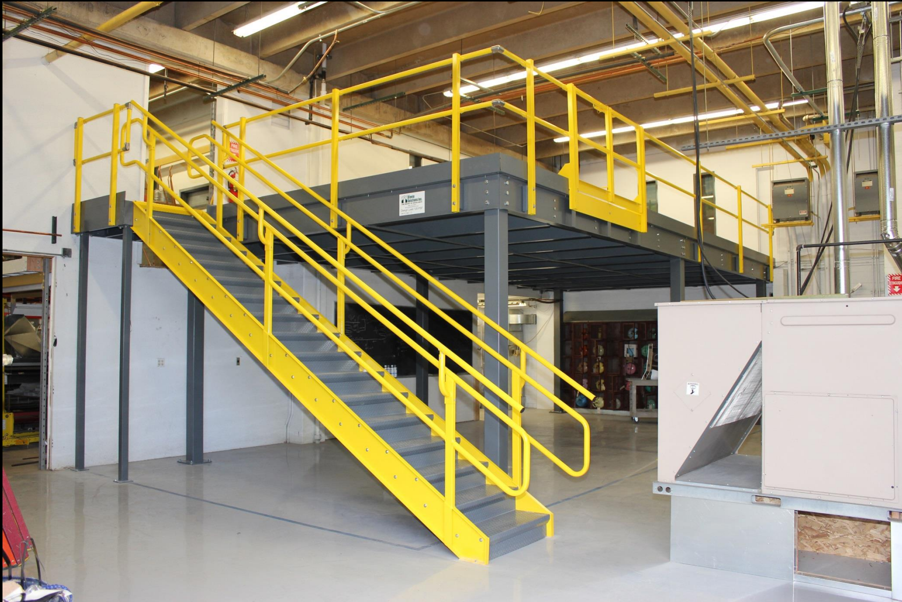
After Photo - Free-Standing Mezzanine
