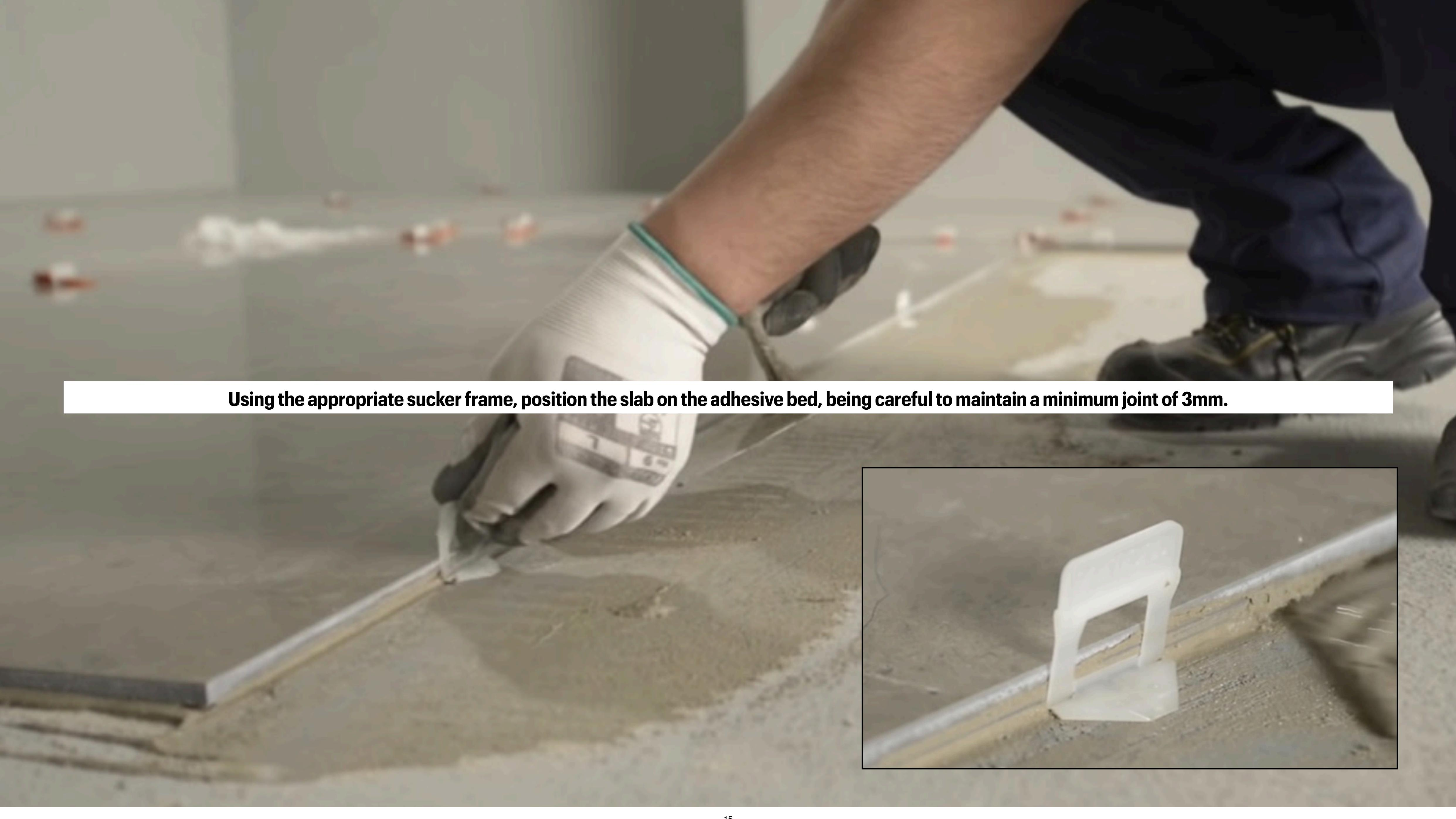
**Using the appropriate sucker frame, position the slab on the adhesive bed, being careful to maintain a minimum joint of 3mm.**
