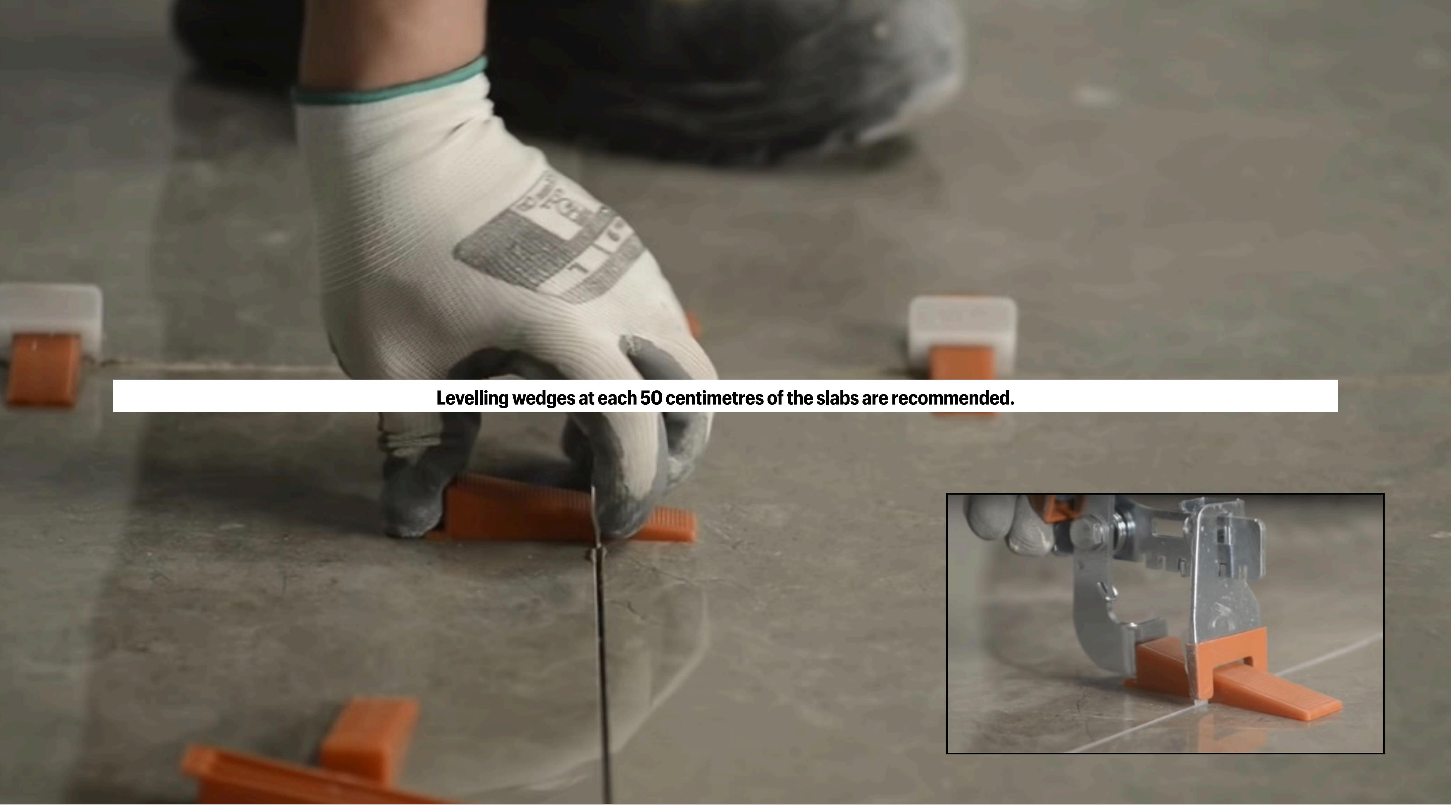
**Levelling wedges at each 50 centimetres of the slabs are recommended.**
