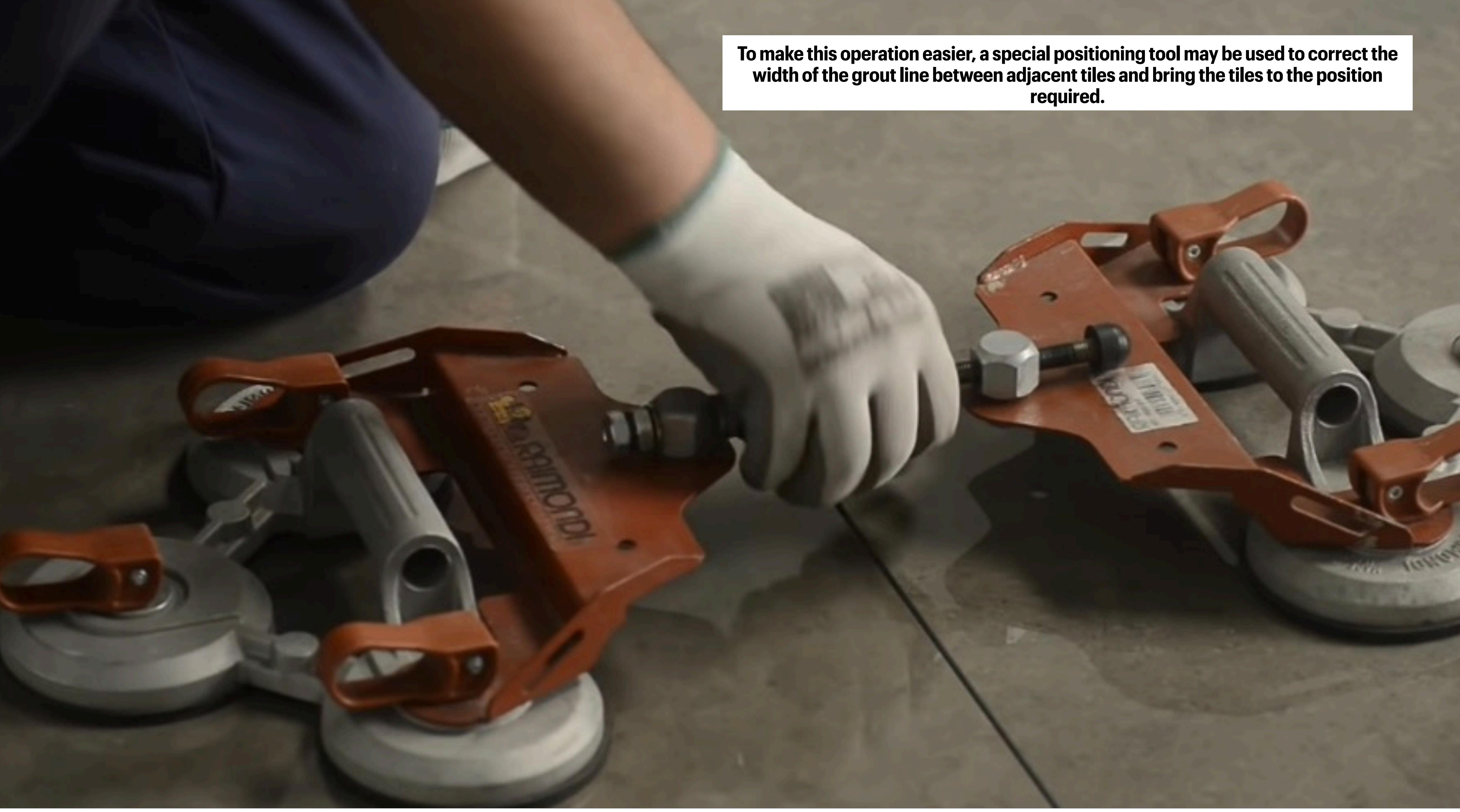
**To make this operation easier, a special positioning tool may be used to correct the width of the grout line between adjacent tiles and bring the tiles to the position required.**
