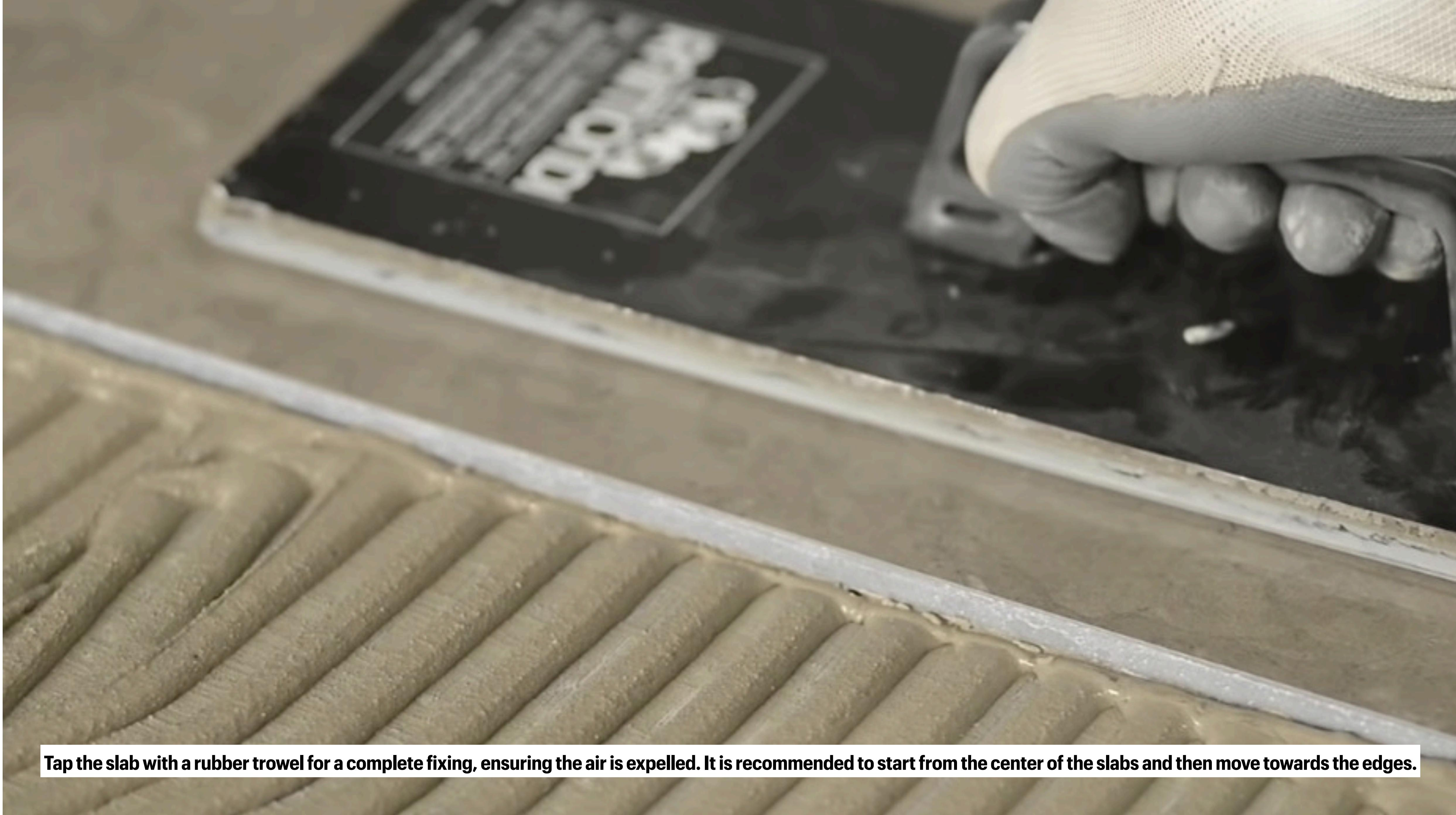
**Tap the slab with a rubber trowel for a complete fixing, ensuring the air is expelled. It is recommended to start from the center of the slabs and then move towards the edges.**
