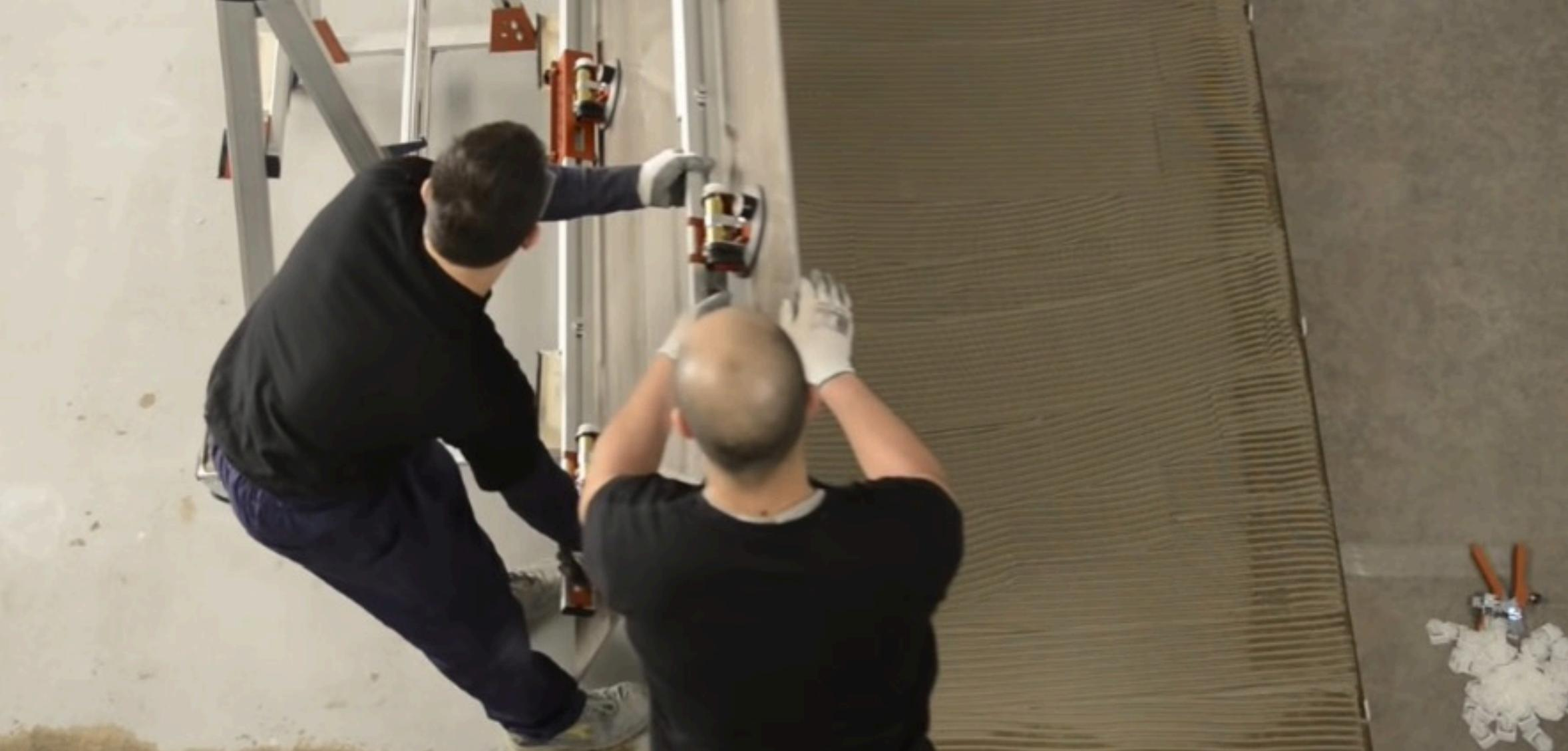
Using the appropriate sucker frame, position the slab on the adhesive bed, being careful to maintain a minimum joint of 3mm.
