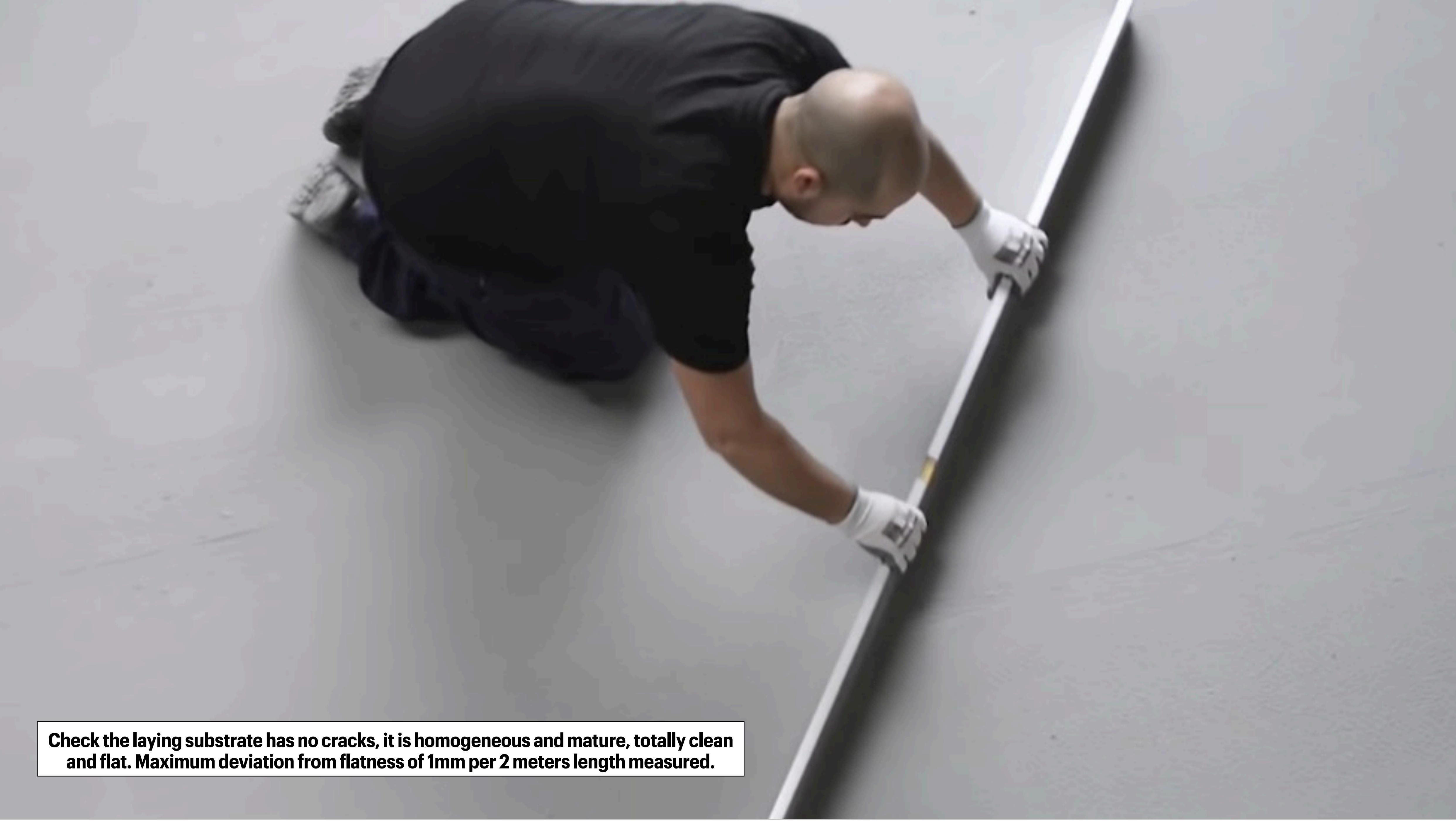
**Check the laying substrate has no cracks, it is homogeneous and mature, totally clean and flat. Maximum deviation from flatness of 1mm per 2 meters length measured.**
